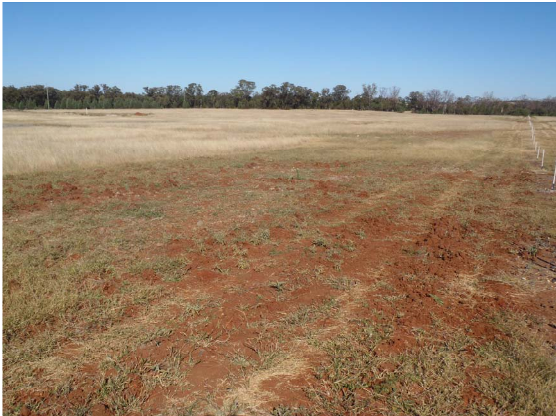
Plate 9 – Ploughing of Cracks in Longwall Panel 1
